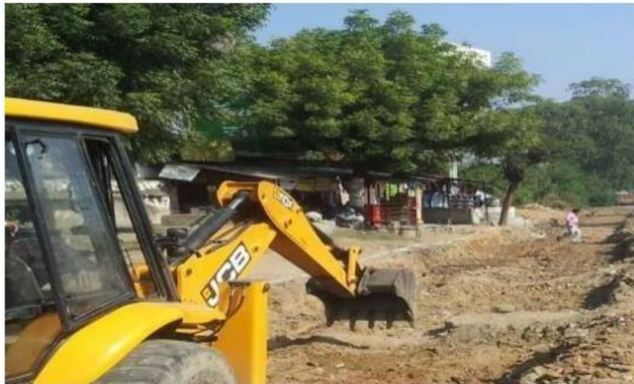
Figure : site clearance
