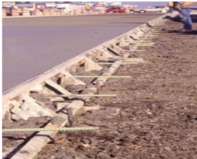
Fig: Steel Form Work for CC pavement Construction
