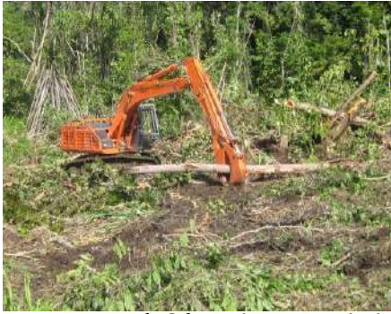
Land Clearing Activities
