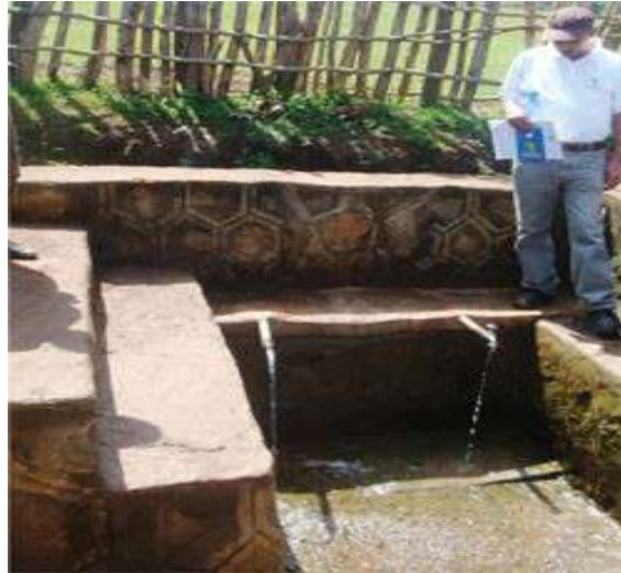
Figure : A protected spring. Note the concrete retention wall with two delivery pipes and the surrounding fence.
