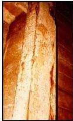
Fig.5.3: Carbonation leads to the general corrosion along the full length of the bar.
