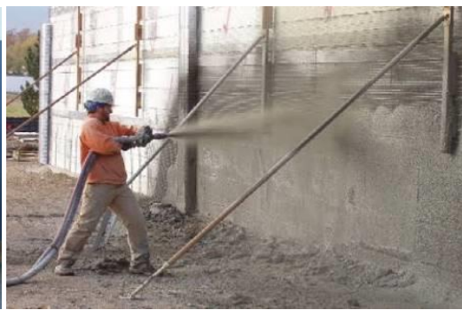
Guniting the prepared surface
