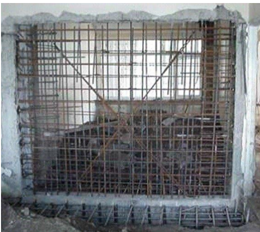
Fig 2: Additional Shear Wall
