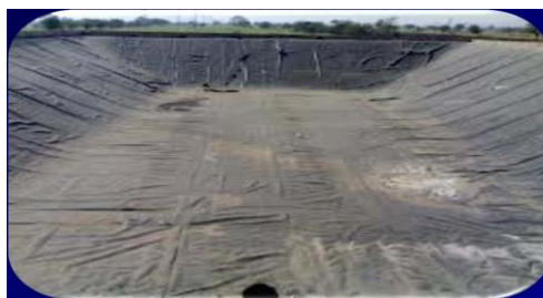
Installation of Geomembranes
