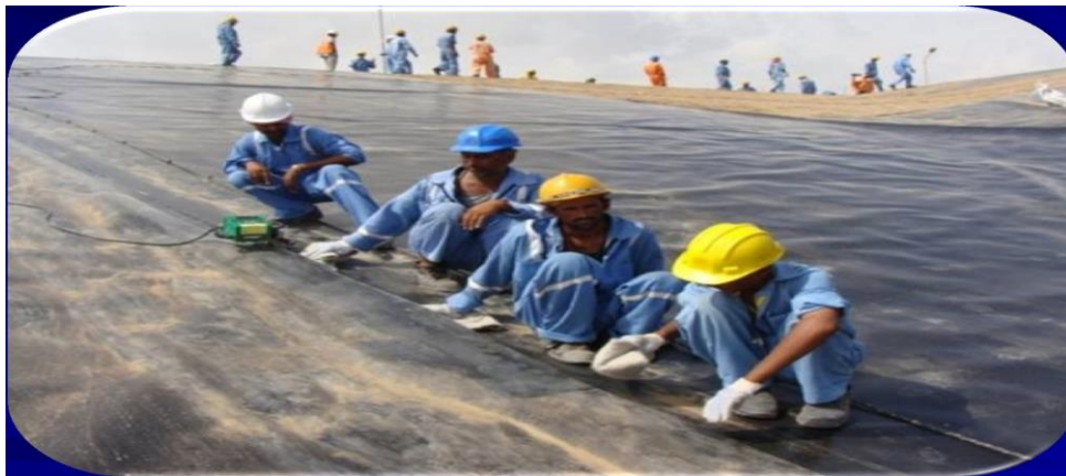
Installation of Geomembranes
