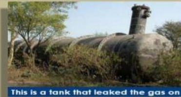
This is a tank that leaked the gas on
