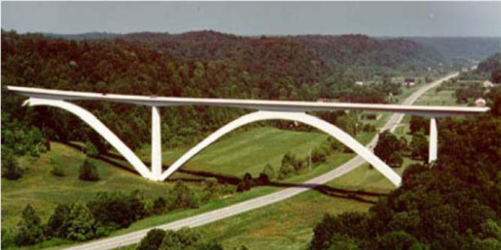
Natchez Trace Parkway Bridge (1994), Tennessee, USA, 502 m span
